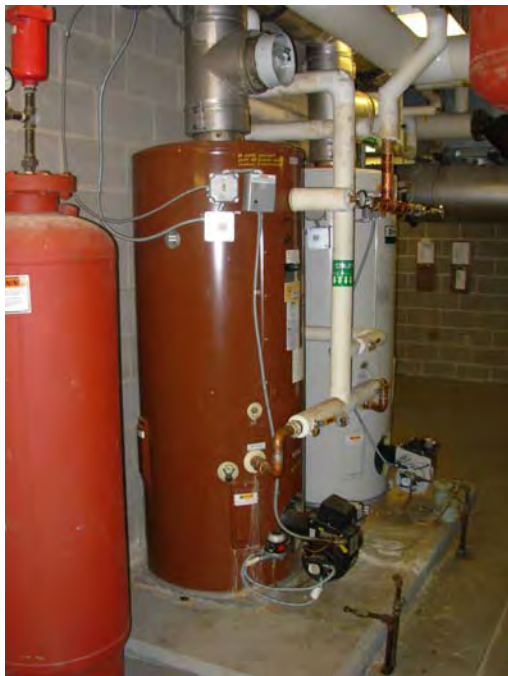
15. Domestic hot water generation tanks
