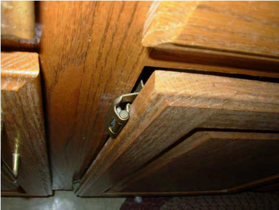
21. Hardware failures and finish wear on most cabinetry sets
