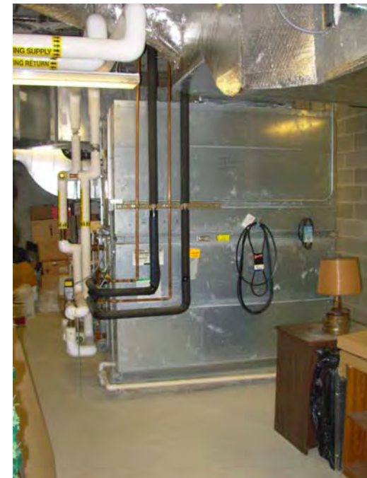
16. Central core HVAC system air handler in basement
