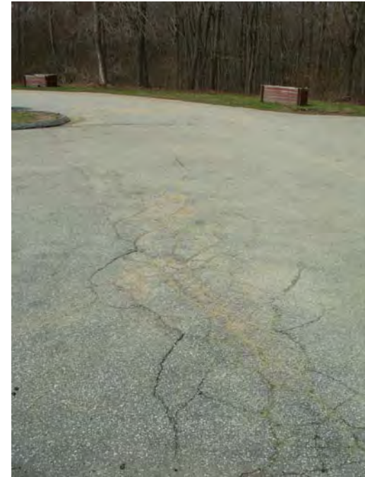
2. Cracking and settlement of asphalt paving
