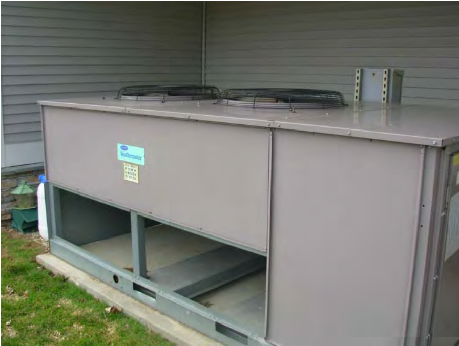
17. Carrier Weathermaster AC condenser unit at rear of building
