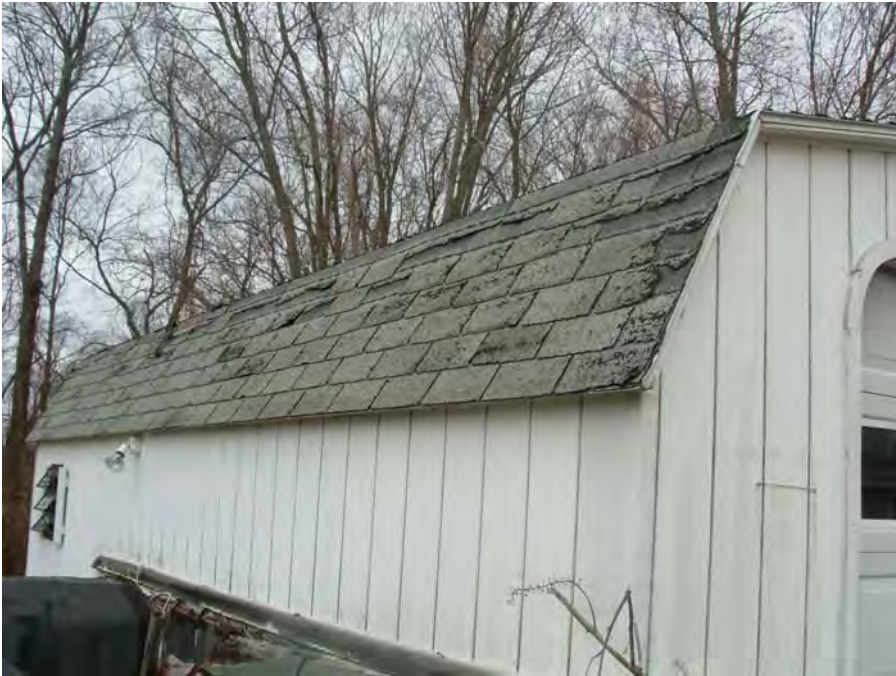
5. Maintenance garage roofing-siding in need of repair
