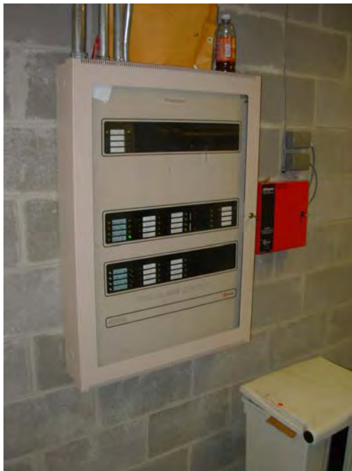
19. Main fire detection - monitoring panel
